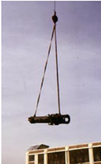
Above, top: Crane beside Patton-McGuyer building. Note roll-off roof observatory in open position on top of building. Middle: Close-up of Patton's observatory. Bottom: Moving the tube assembly to the truck for transport. Above right: Bob Howe and the crane operator examine Ralph C. Patton's 12-inch reflector. Photos from Skyscrapers collection.
