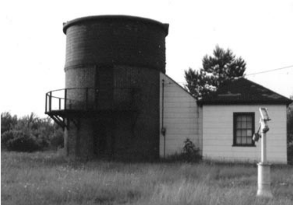
Top: October 6, 1956. A good crowd of visitors at the third annual AstroAssembly convention. A nice collection of telescopes as well. Looks like the Trustees needed to conduct a little repair work on the anteroom roof. Skyscrapers collection. Bottom: Another photo from 1956. The mount on the right, still out in the courtyard as of this writing, is for the 6-inch refractor. Notice that the trees are encroaching. Skyscrapers collection.
