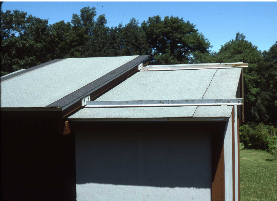
L) The sliding door and roof panel in place. R) the crank and chain apparatus connected to the under-floor gear system
