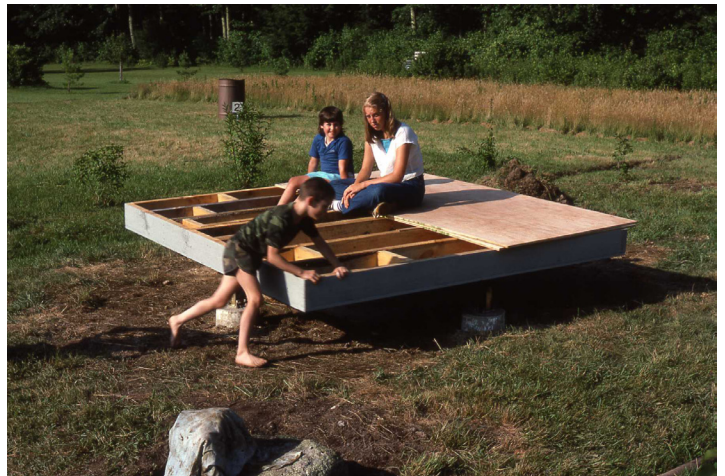
I pre-fabricated and pre-painted the walls in the shade of an elm tree. Then, with the help of a neighbor, I attached the walls to the 8' x 8' rotating floor.
