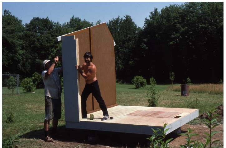
I pre-fabricated and pre-painted the walls in the shade of an elm tree. Then, with the help of a neighbor, I attached the walls to the 8' x 8' rotating floor.
