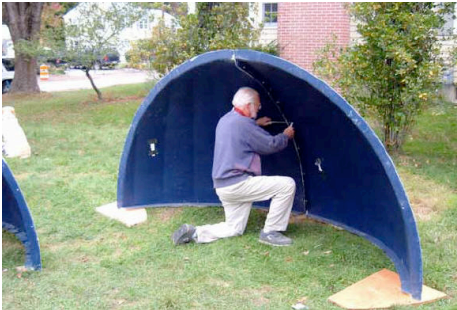
ay, Oct 11 - Dave's been working for weeks refinishing the dome. Now it's time to assemble the dome quadrants.
