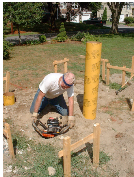
I'd been cautioned that the foundation layout is critical. So I laid out batter boards galore.
