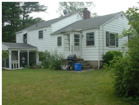
Rear porch demolished.
