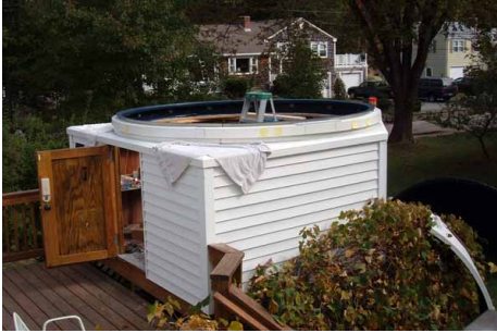
Thursday, Oct 10th - The dome support ring's been assembled over the base ring. Lookin' good.
