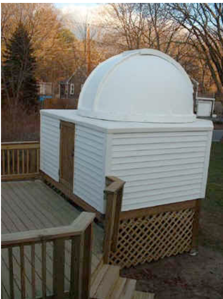
January 9, 2007. The structure is finally complete - except for plantings which will have to wait until spring. The 14" is already
