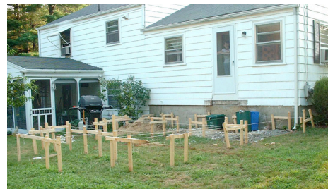
I'd been cautioned that the foundation layout is critical. So I laid out batter boards galore.
