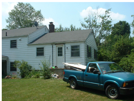
Rear landing demolished.
